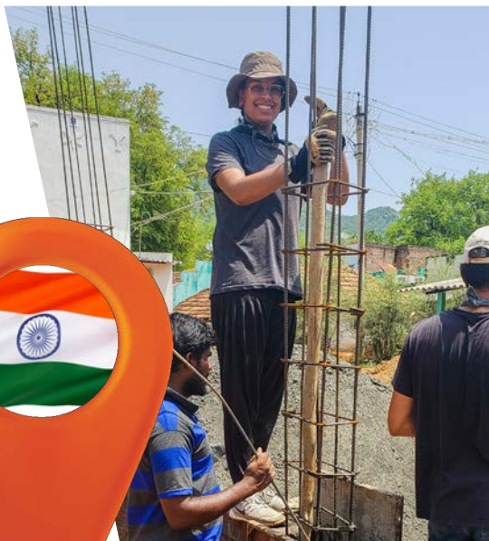
Left: PUC India Team building the foundation of a children's library
